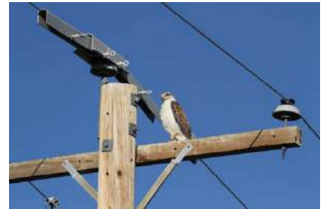
▲ A Ferruginous hawk rests on a 3-phase pole protected with a conductor cover on the center pin.
