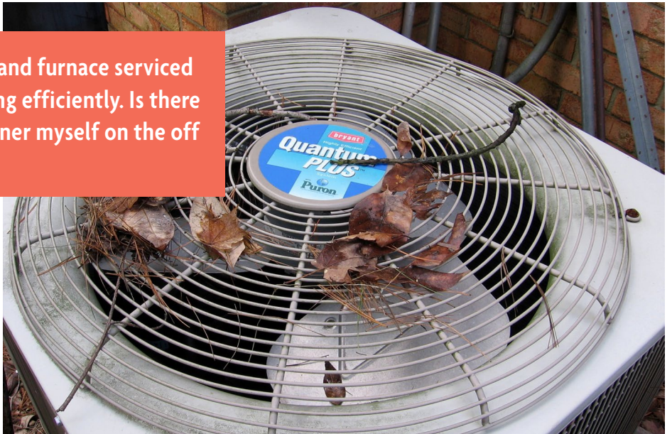
▲ Clean leaves and other debris from the top of the central air conditioner unit even though many will blow away by themselves when the unit starts. Photo by James Dulley.
