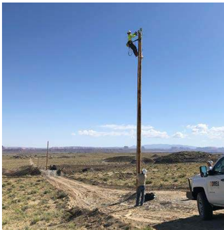
▲ A DMEA crew works to wire poles for Light Up Navajo.
