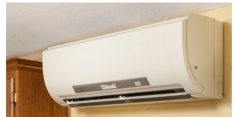
▲ Ductless heat pumps have increased in popularity significantly over the past 10 years. They are a great solution for homes that do not have existing ductwork. Photo courtesy of Bonneville Power Administration.
