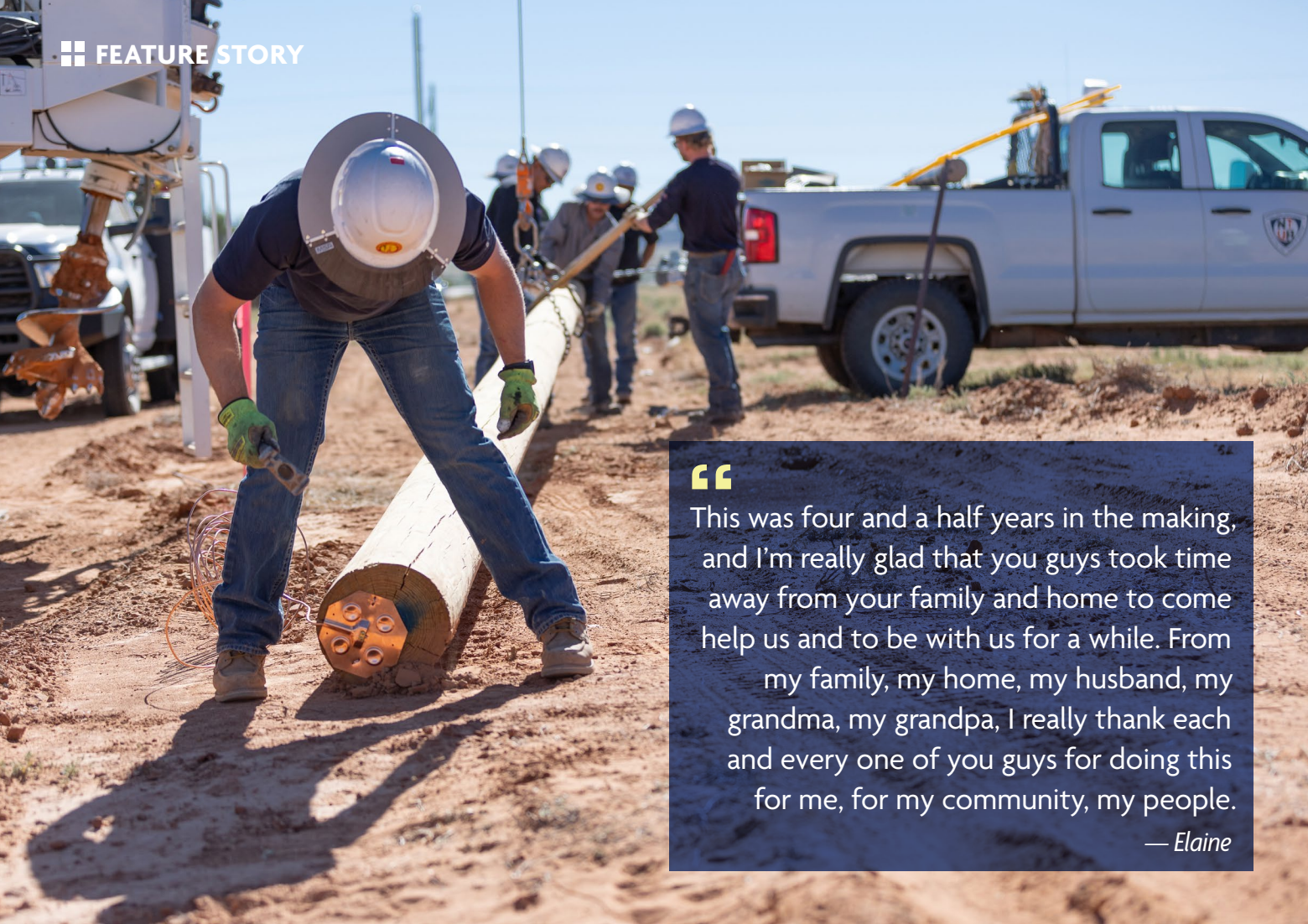
▲ A Colorado linecrew prepares a power pole before it is set into the ground in Chinle, Arizona, in June.
