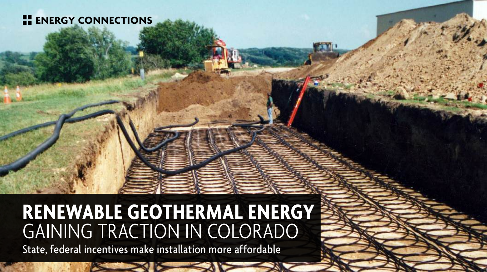
▲ A crew installs the in-ground water circulation loops for a ground-source heat-pump system.
