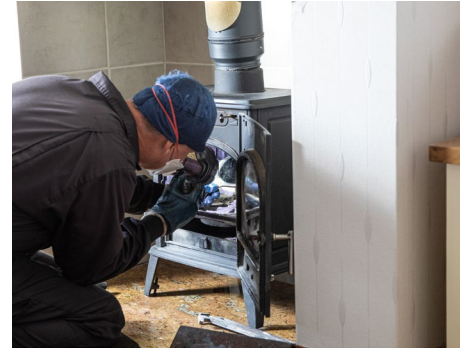
▲ Make sure a chimney sweep does a camera inspection and shows you the video.
