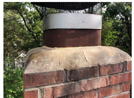
▲ Check your chimney crown for loose parts needing repair.
